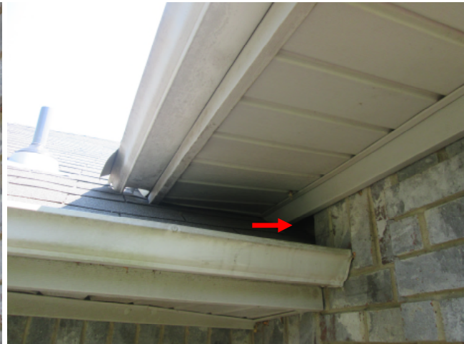
Opening in brick veneer.
