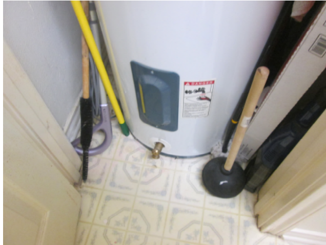
Missing safety drain pan.
