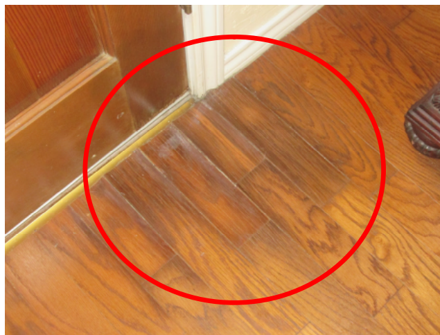
Previous moisture damage to wood floor.
