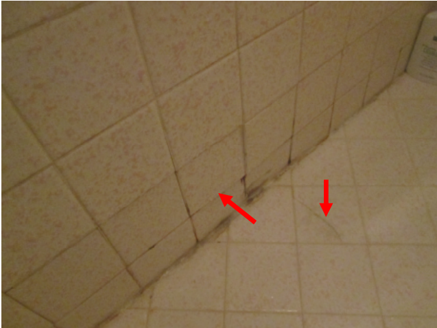
Moisture damage to shower wall and cracked tile.
