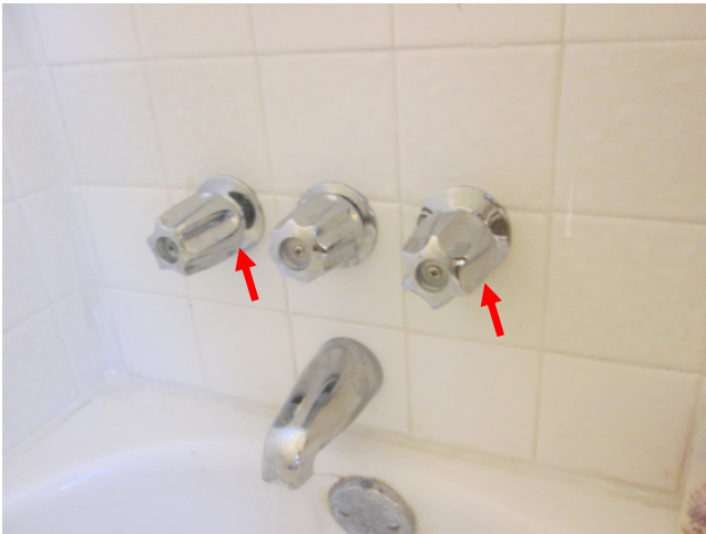
Tub faucet valves are leaking.
