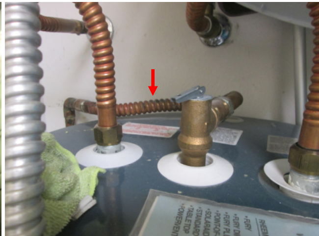
Pressure relief pipe routed in flex copper.
