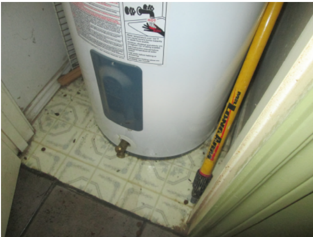
Missing safety drain pan.
