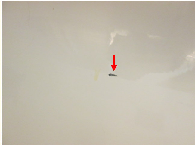
Chip in tub porcelain coating.
