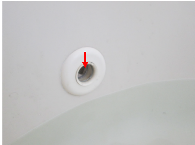
Missing jet insert.
