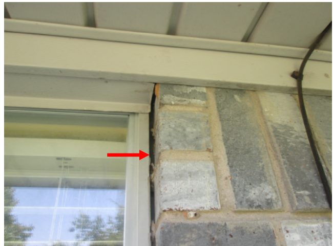
Separation between window trim and brick veneer showing signs of previous movement.
