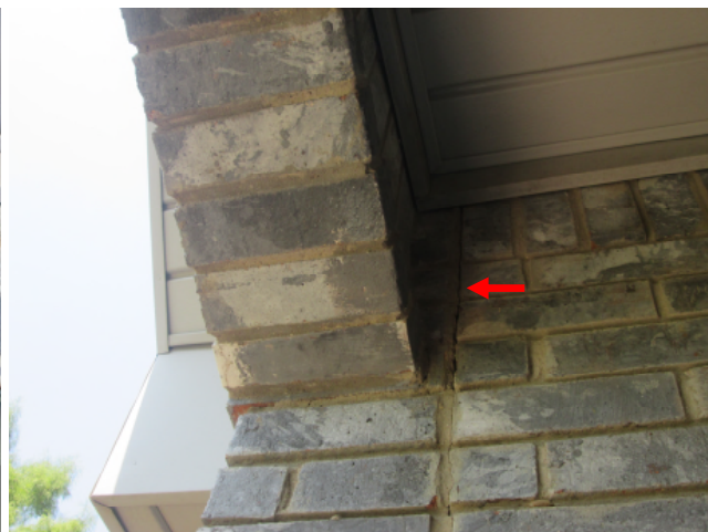
Mortar openings in brick veneer.
