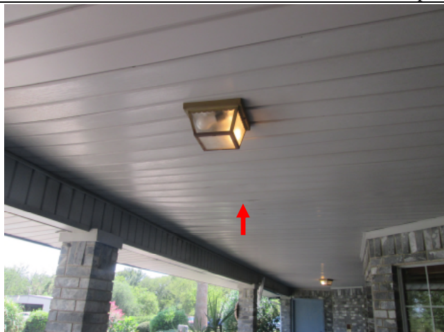
Loose soffit above back patio.
