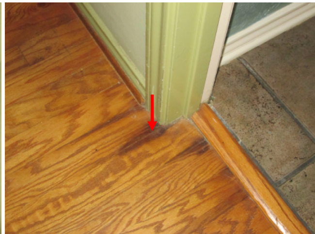
Previous moisture damage to wood floors.
