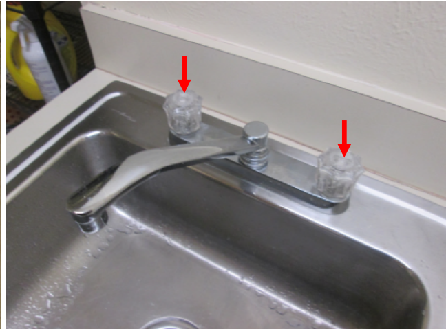
Hot and cold valves are reversed.
