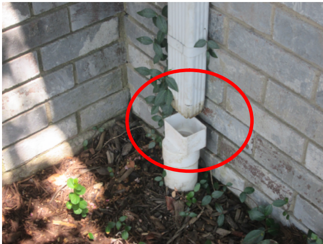
Disconnected gutter down spouts.
