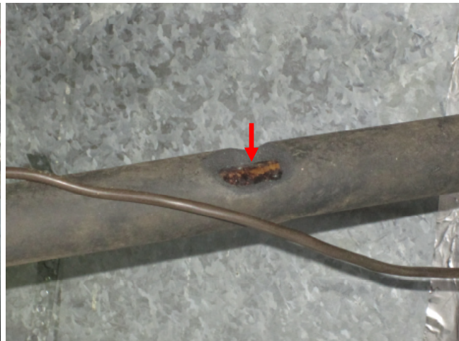
Suction line needs insulated or sealed.
