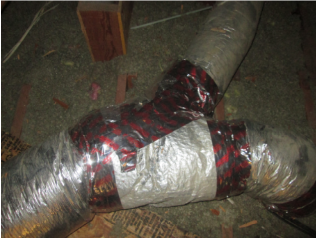
Duct work taped in various places
