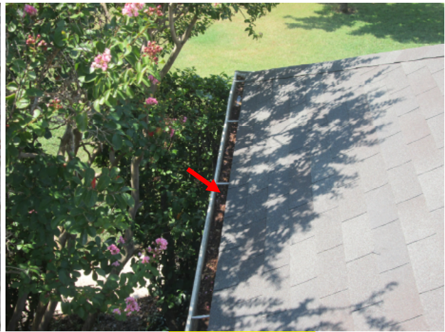
Debris in gutters.
