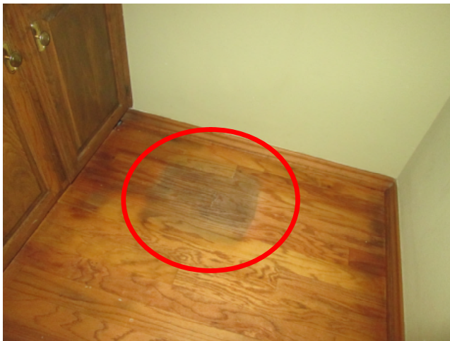
Previous moisture damage to wood floors.
