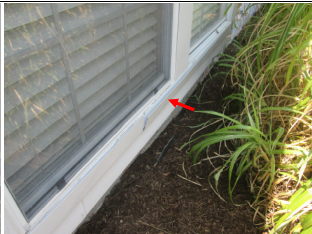
Loose metal window trim wrapping.
