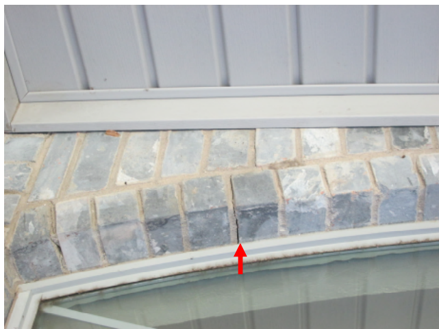
Mortar openings in brick veneer.
