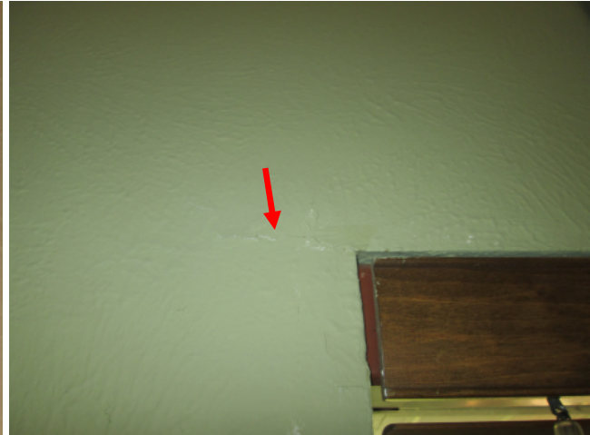
Various stress cracks above windows on south side of house.
