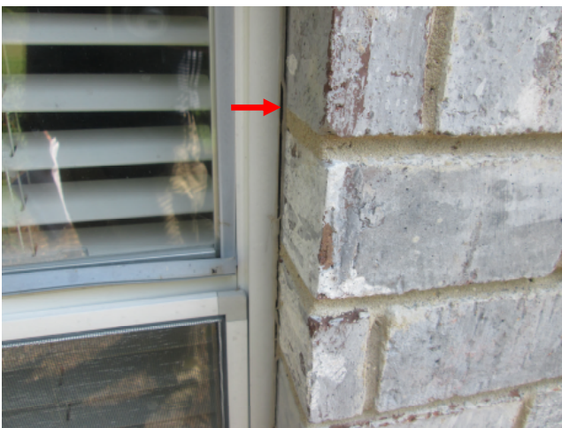
Touch up caulking needed around windows.
