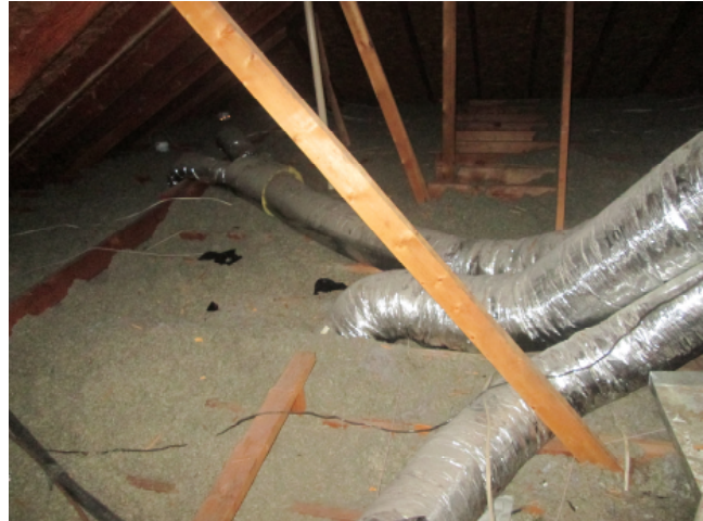
Duct work not suspended off insulation.
