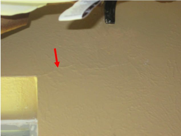
Various stress cracks above windows on south side of house.
