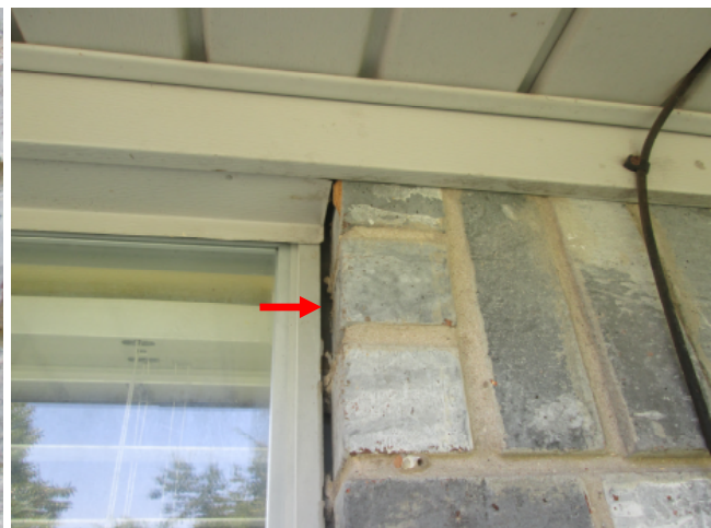
Window showing signs of previous movement.
