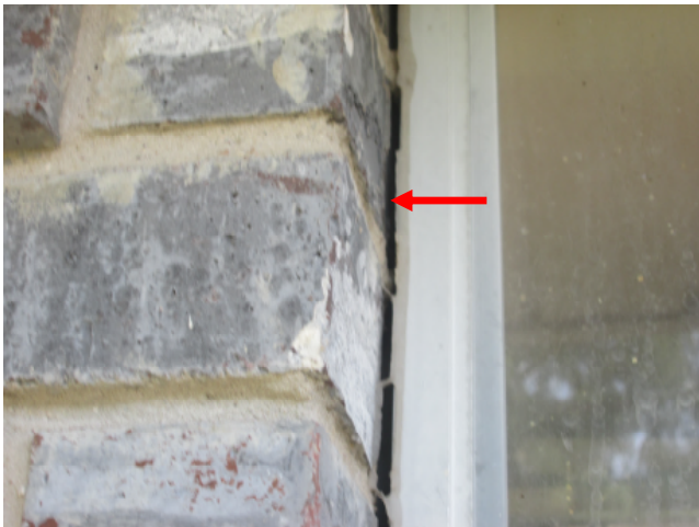
Separation between window trim and brick veneer showing signs of previous movement.
