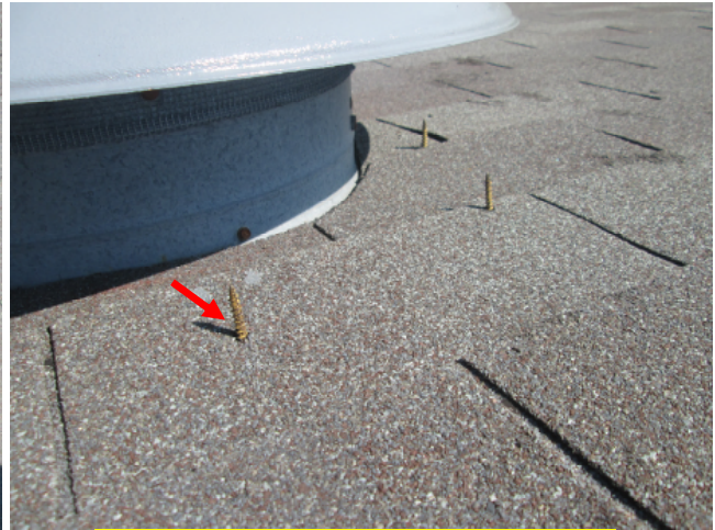
Screws sticking out through the roof.
