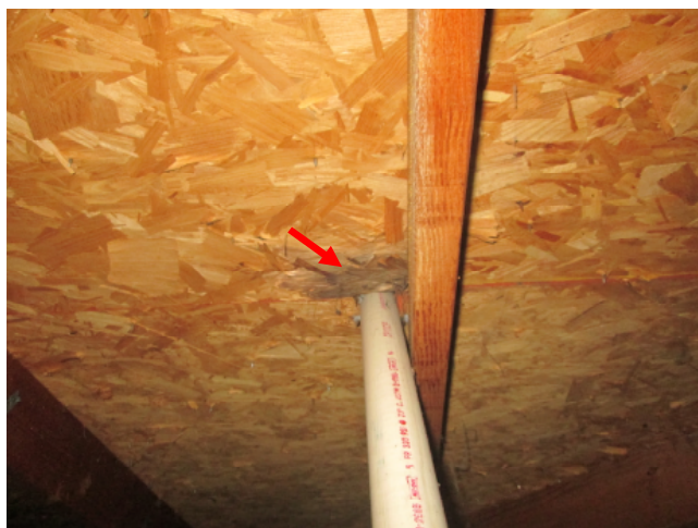
Previous moisture damage around vent pipe.
