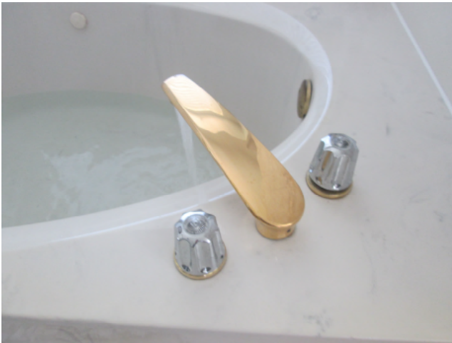
Loose tub faucet, stiff cold water valve and hot valve will not turn off.
