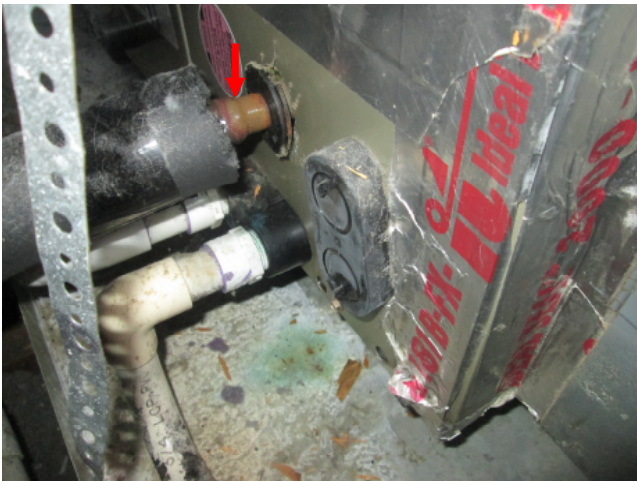
Suction line needs insulated next to evaporator coil.
