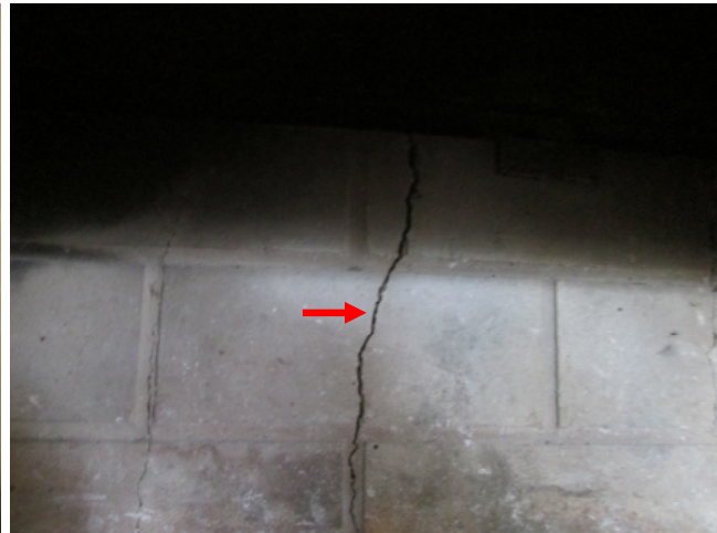
Crack in back of firebox.
